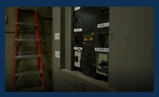
**ORIGINAL ELECTRICAL PANEL** The main electrical panel is outdated and becoming difficult to repair. It does not meet current code standards.
